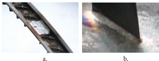
Figure 6. Guide vanes repair: a – blade dismantling place after metalworking; b – a blade after soldering
