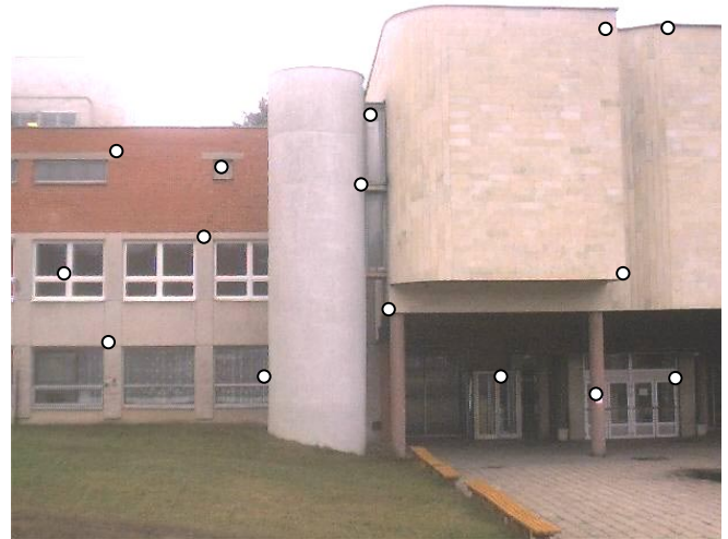
Fig 4. Outdoor test field
