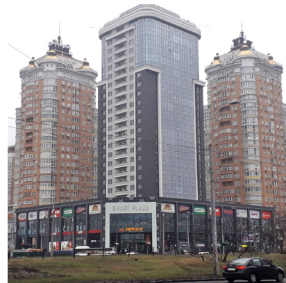
Figure 6. Commercial use of a part of a residential building
