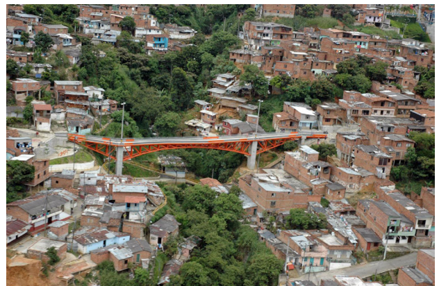
Figure 4. The "De la Paz y la Cultura" pedestrian bridge linking the La Francia and Andalucía neighborhoods (source: Universidad EAFIT, 2013)
