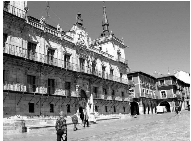
Fig. 2. A façade in Leon, northern Spain
