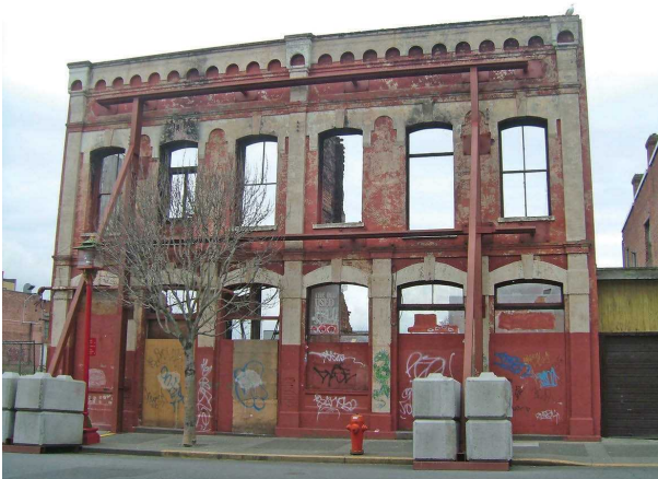
Fig. 5. "Dead" façade in Victoria, British Columbia, Canada
