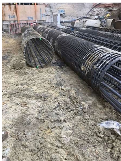
Figure 1. Prefabricated steel piles on the case site (taken by the authors)
