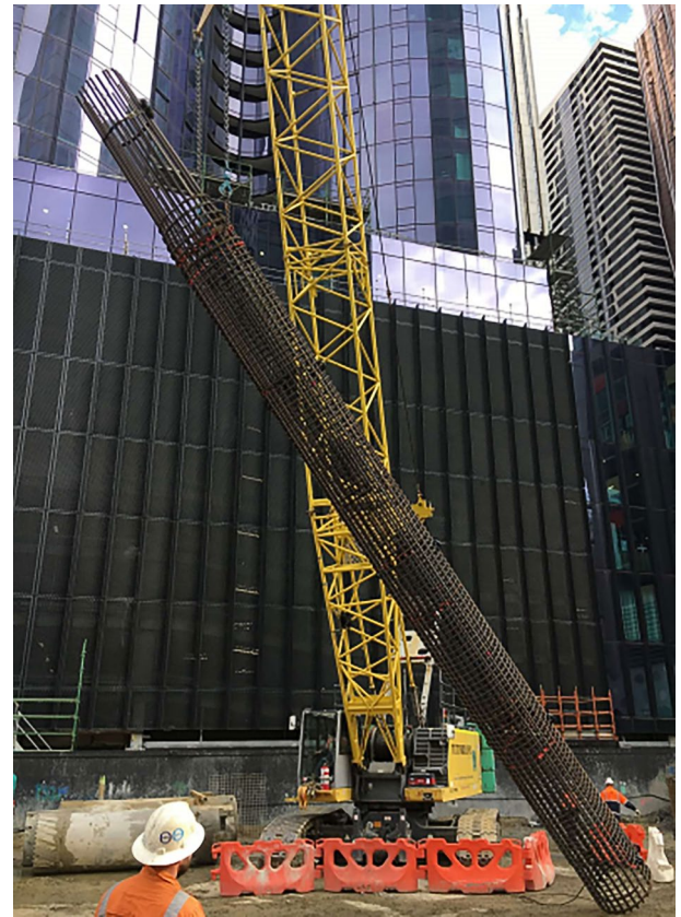
Figure 4. Lifting of one of the longest pile sections
