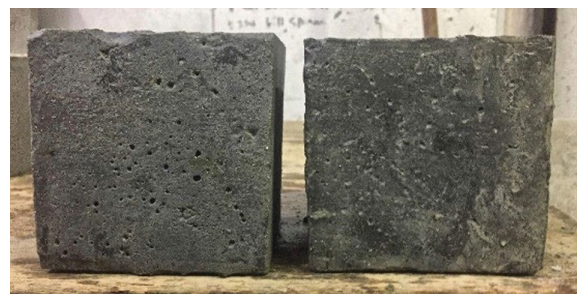
Figure 18. Appearance investigation after 28 days of immersion in MgSO 4
