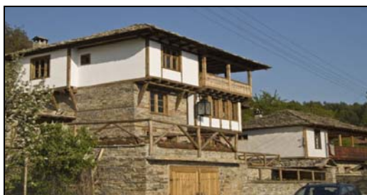
Fig. 4. Traditional Bulgarian building
