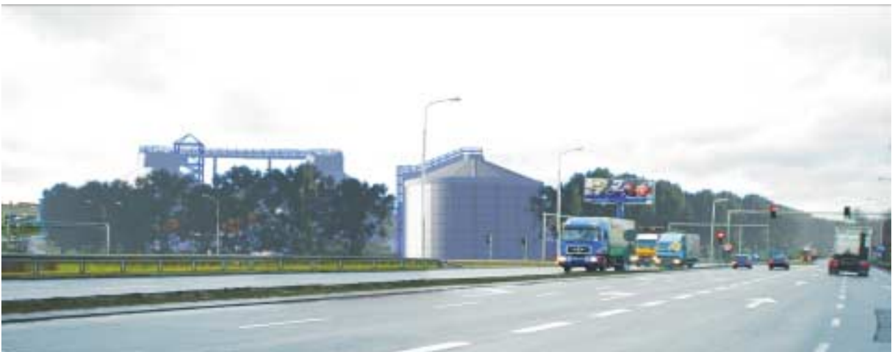
Fig 2. Computer visualisation of water purification plant LOS, Poznan (Poland), from the viewpoint of a car driver (Plant design: Aqua Poznan)
